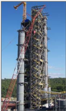
Pre-heater tower and stack
