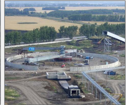
Raw material storage
