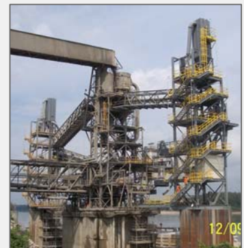
Barge loading facility
